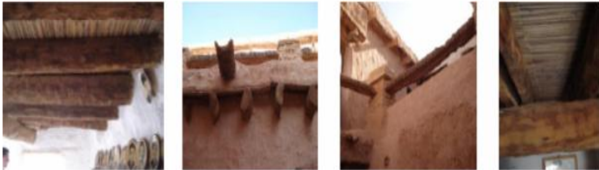
Fig. 4. Various uses of palm trees: beams, gutters, fences, and false ceilings 29 .
