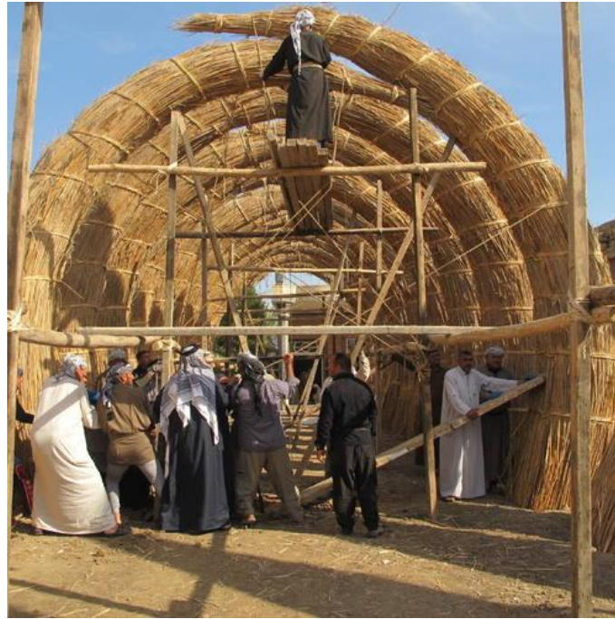
Fig. 7. Construirea unui mudhif. Sursa: https://twitter.com/UNESCOIraq/status/754758295047602176/photo/3
